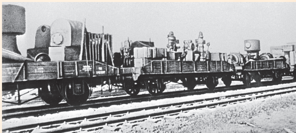
Train with equipment of evacuated plant goes to East. 1941
