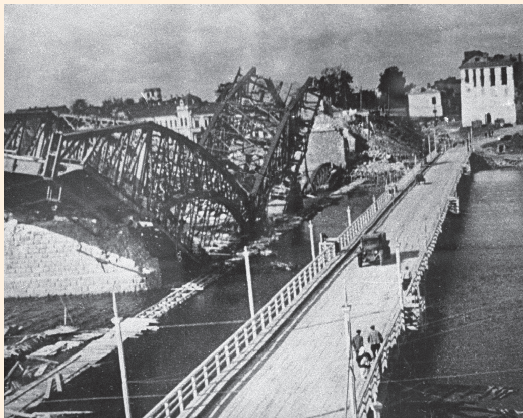
Bridge at suburb of Pskov city, 1944
