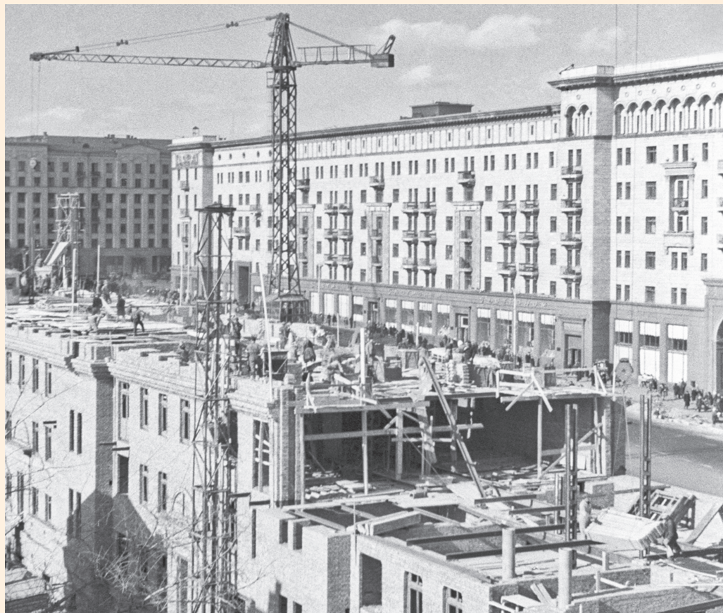
Construction of dwelling-houses in Gorky Street in Moscow. 1946
