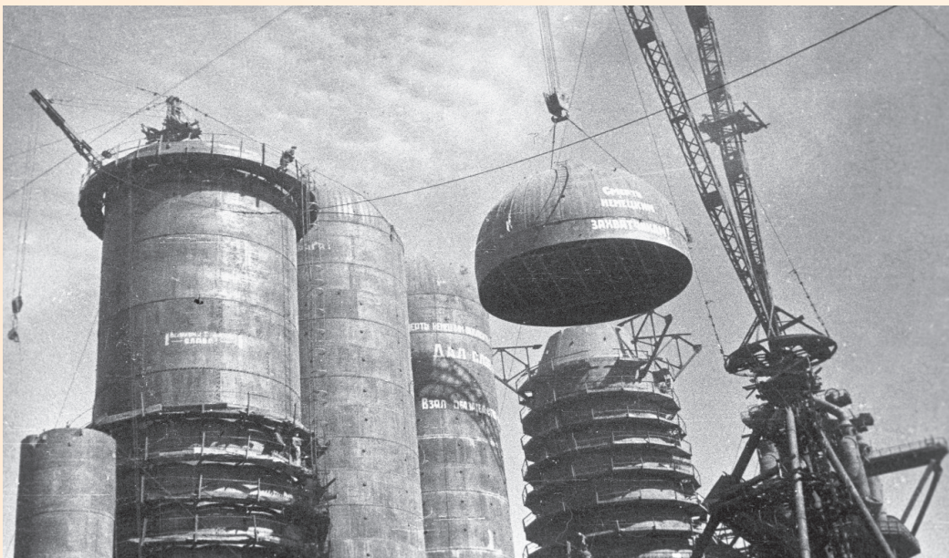
Construction of the sixth blast furnace in Magnitogorsk. 1943
